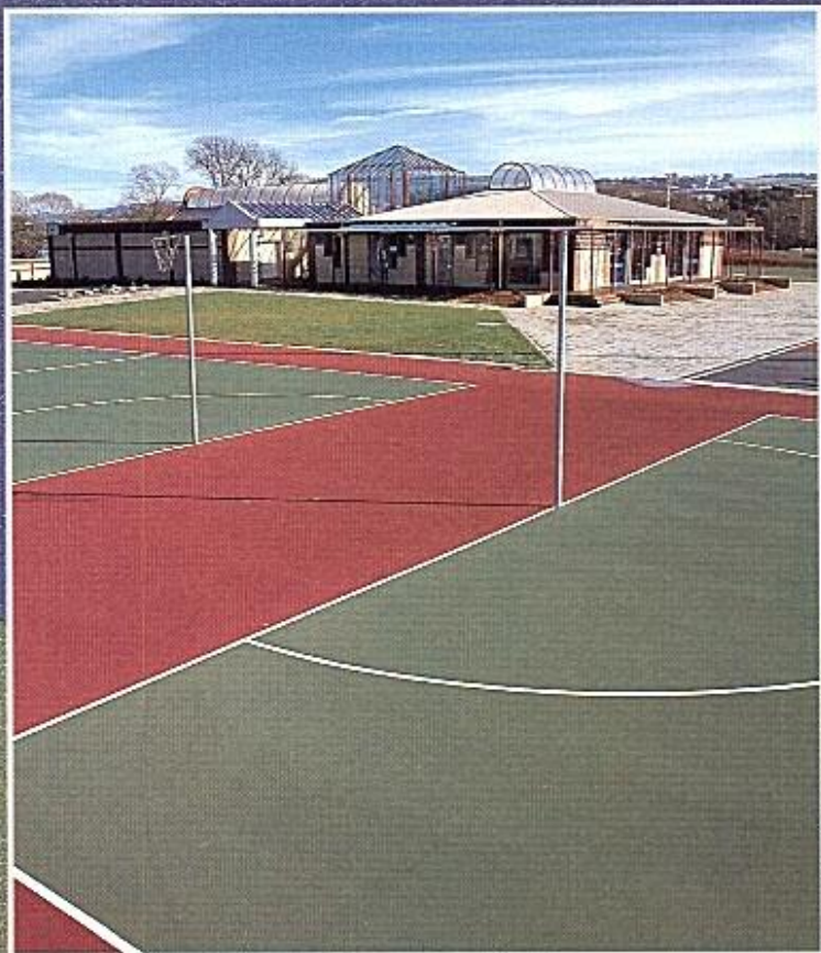
Launceston Netball Centre
