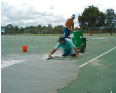
Photo 2 - Repairing depressions in court surface
